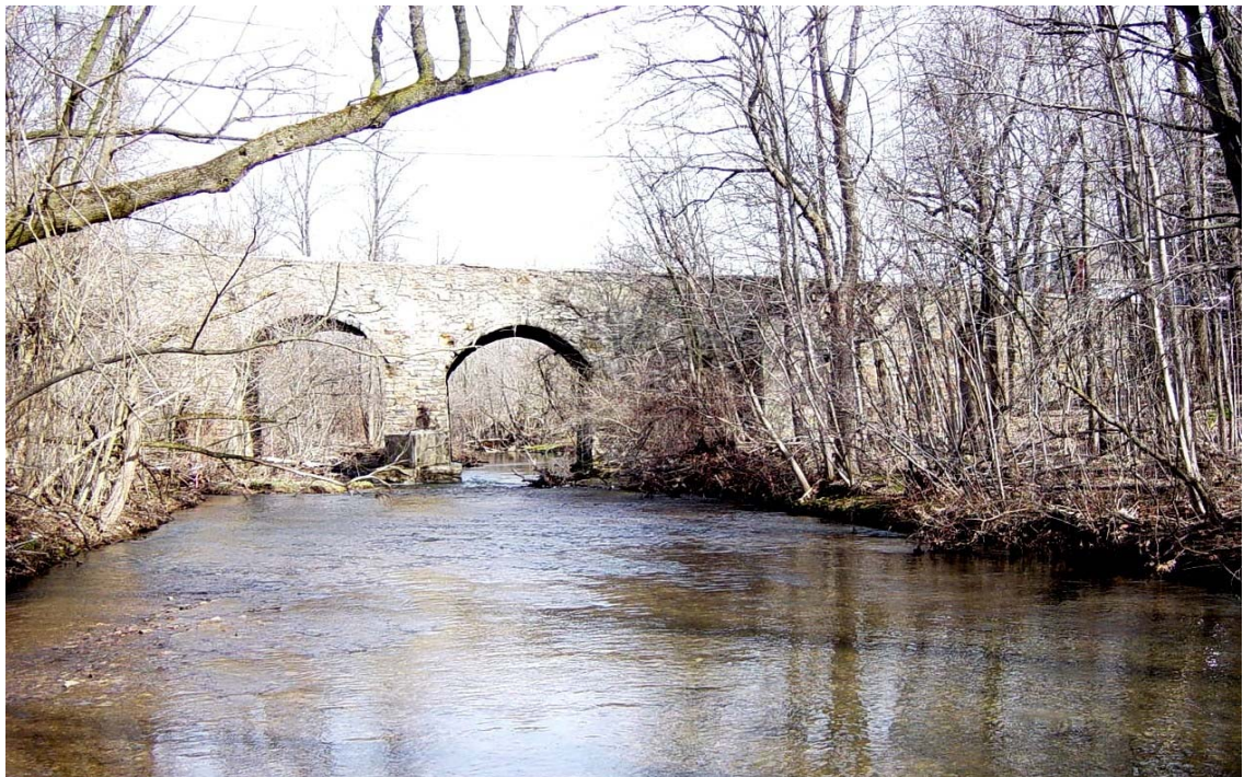
Centennial Bridge over the Saucon Creek, the Region's only Nationally-Registered Historic Site
