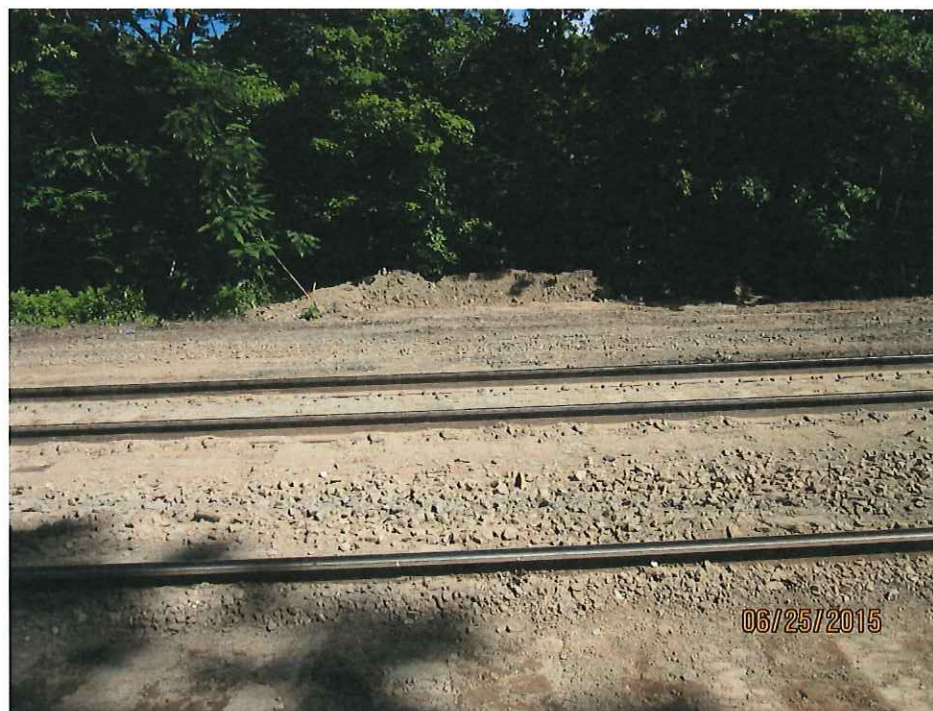
3-4. Looking north across the railroad bed at the washout location, showing soil and rock material deposited across both sets of tracks. Note large pile of soil and rock pushed up by machinery on the far (north) side of the rail bed.
