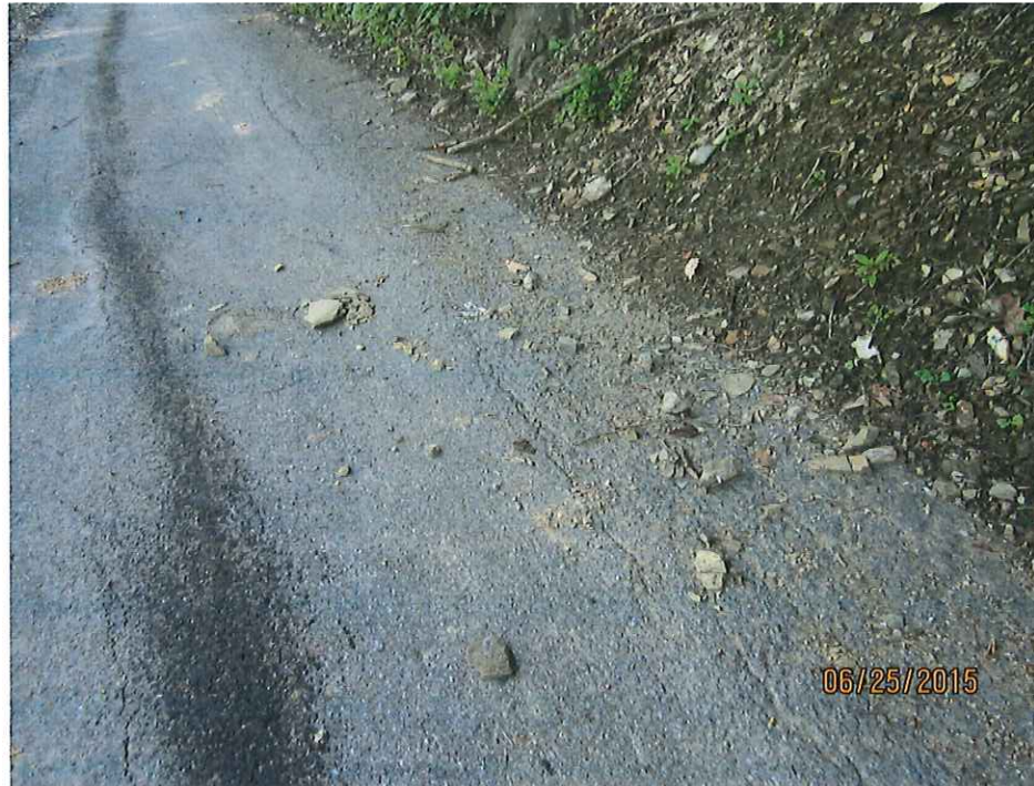
2-3. Close-up of small amount of outwash onto road surface just upslope of area of undermining.
