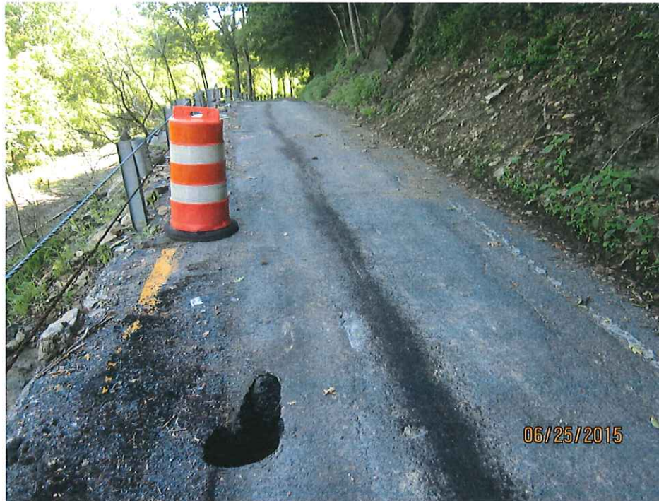
2-1. Overall view of Riverside Drive in the area of undermining, showing hole in road surface (foreground) and small amount of outwash onto roadway (background).
