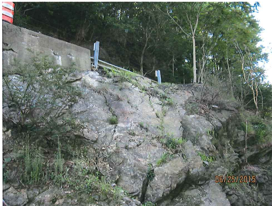
2-6. Close-up of outcrop of competent bedrock on west side of fracture zone.
