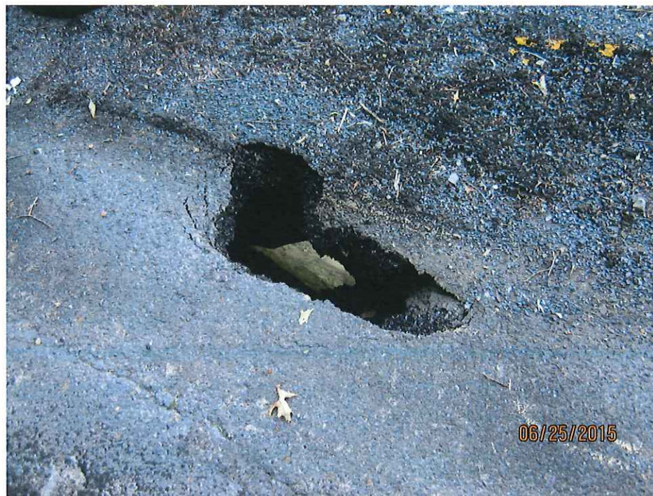
2-2. Close-up of hole in road surface, showing that it extends to daylight below.
