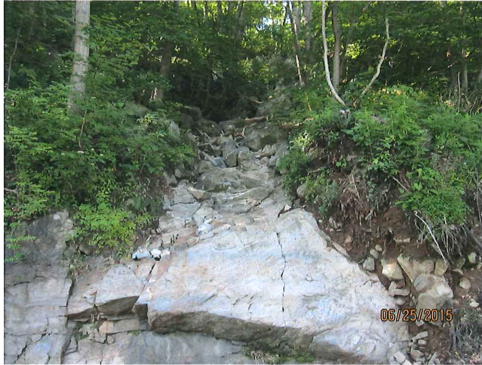
3-2. Looking south from Riverside Drive at the washout location, showing the eroded channel on the slope heading southward.
