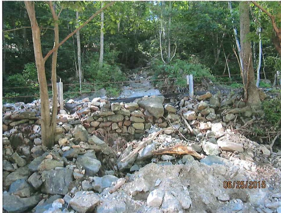
3-3. Looking south from the railroad bed across Riverside Drive at the washout location, showing soil and rock material deposited on the north bank of the roadway.
