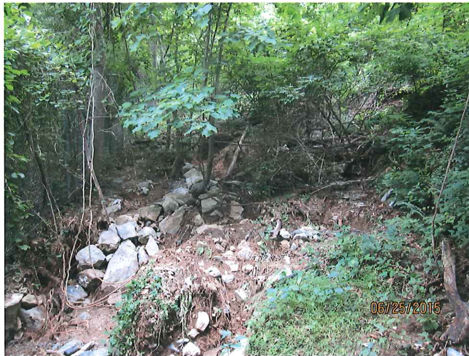
3-14. View downhill of the concrete "sluice", showing soil and rock material eroded by stormwater runoff coming from north slope road.
