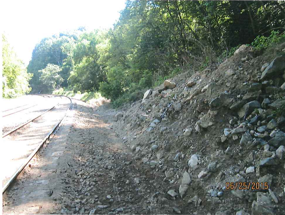
3-5. Looking east along juncture of railroad bed and road bank at outwash location, showing soil and rock material deposited.
