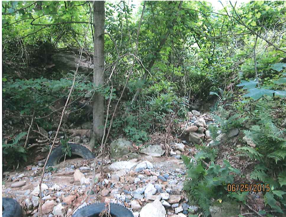
3-15. View downhill of second runoff location, showing soil and rock material eroded by stormwater runoff coming from north slope road.
