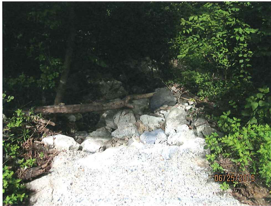
3-12. Close-up of end of concrete sluice and beginning of natural swale on the north slope.
