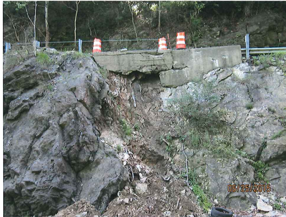
2-4. View of northern bank of roadway at undermined area. Note outcrops of competent dolomite bedrock on either side of undermining and concrete wall anchored to competent bedrock and spanning fracture zone of weathered bedrock.
