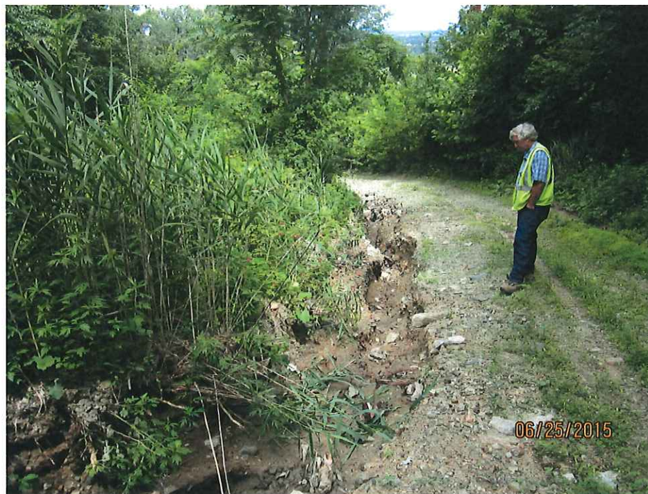
3-8. On the IESI landfill property, looking north along entrance to north slope road, showing erosion channel in road bed cause by stormwater runoff.
