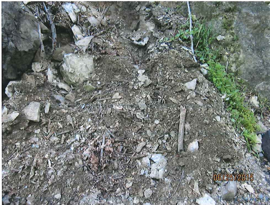
2-8. Close-up of soil and soft rock material eroded from the fracture zone and lying on the railroad bed at the base of the roadway bank.
