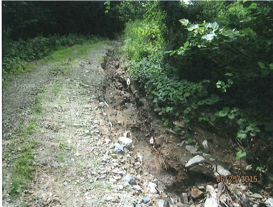
3-9. Close-up of erosion channel on north slope road on IESI property.
