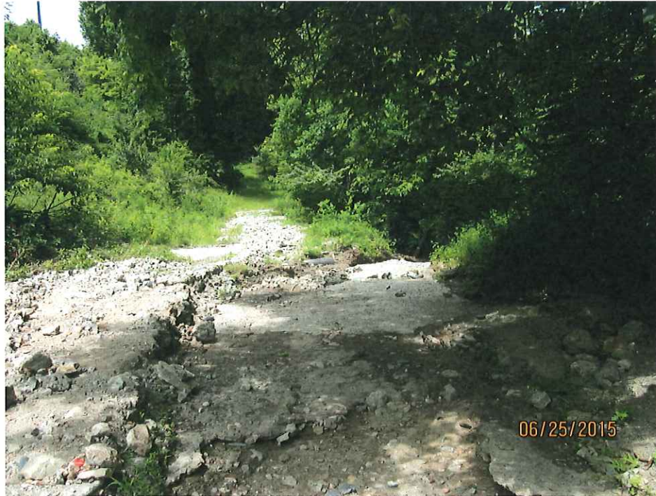
3-11. Looking west along western leg of north slope road, showing beginning of concrete "sluice" which directs stormwater runoff to the north toward a natural swale on the north slope.
