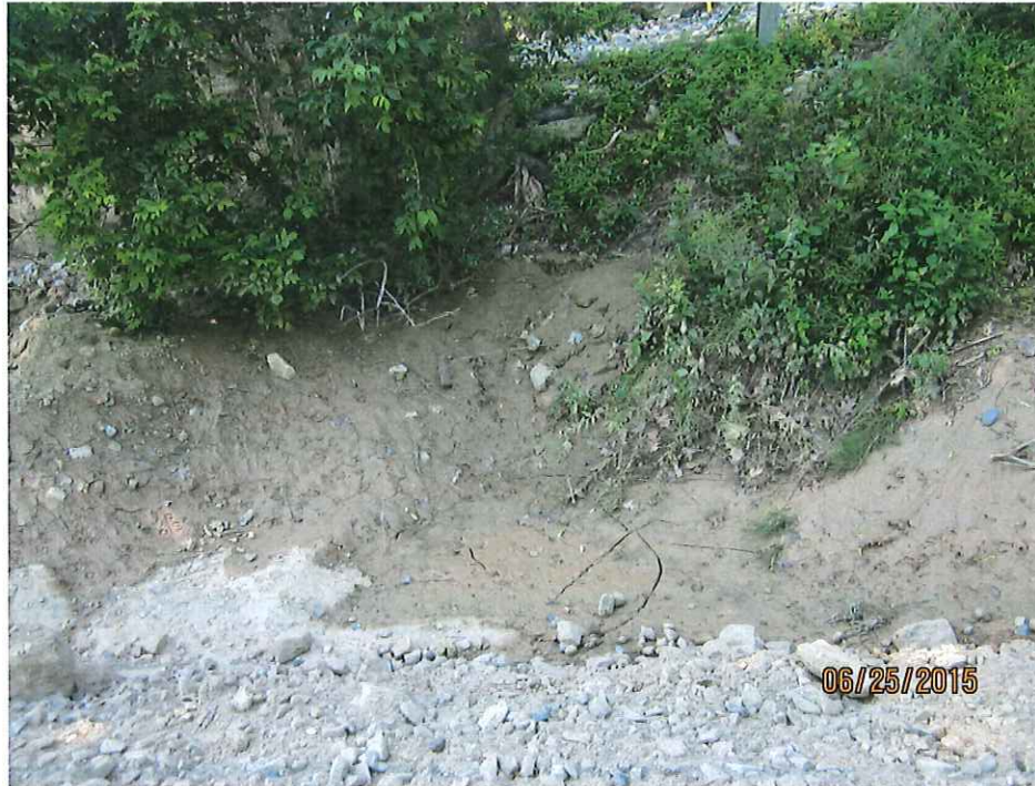
3-7. Close-up of “sump” in ditch along rail bed at bottom of roadway bank. This is opposite the location of the hazard markers on Riverside Drive and may indicate the presence of a culvert or inlet at this location.
