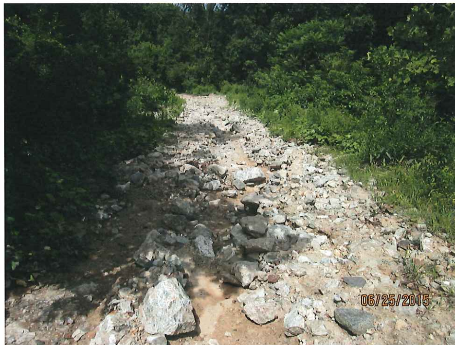
3-10. Looking east along western leg of north slope road, showing rock material deposited by stormwater runoff.
