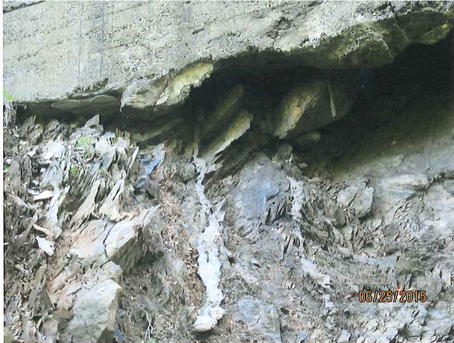
2-7. Close-up of fracture zone in bedrock and undermining of concrete wall constructed to span it. Note thin-bedded and highly weathered nature of the bedrock in the fracture zone.
