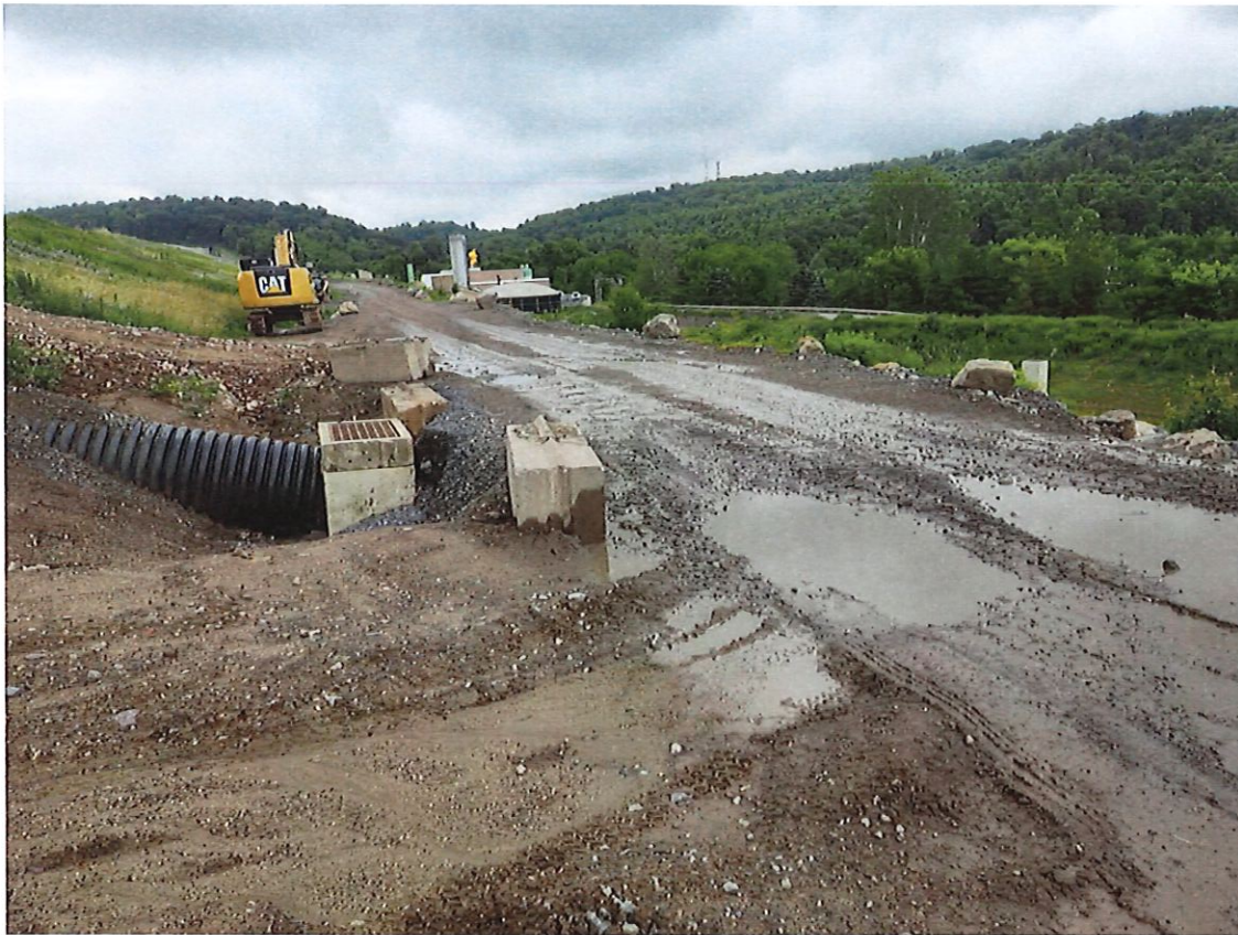
Inlet box and 30-inch HDPE pipe at bottom of the stormwater drainage channel north of Sedimentation Pond 4.
