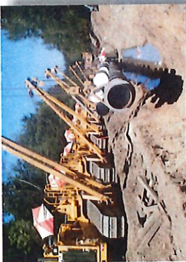
Inspection and repair of coating
