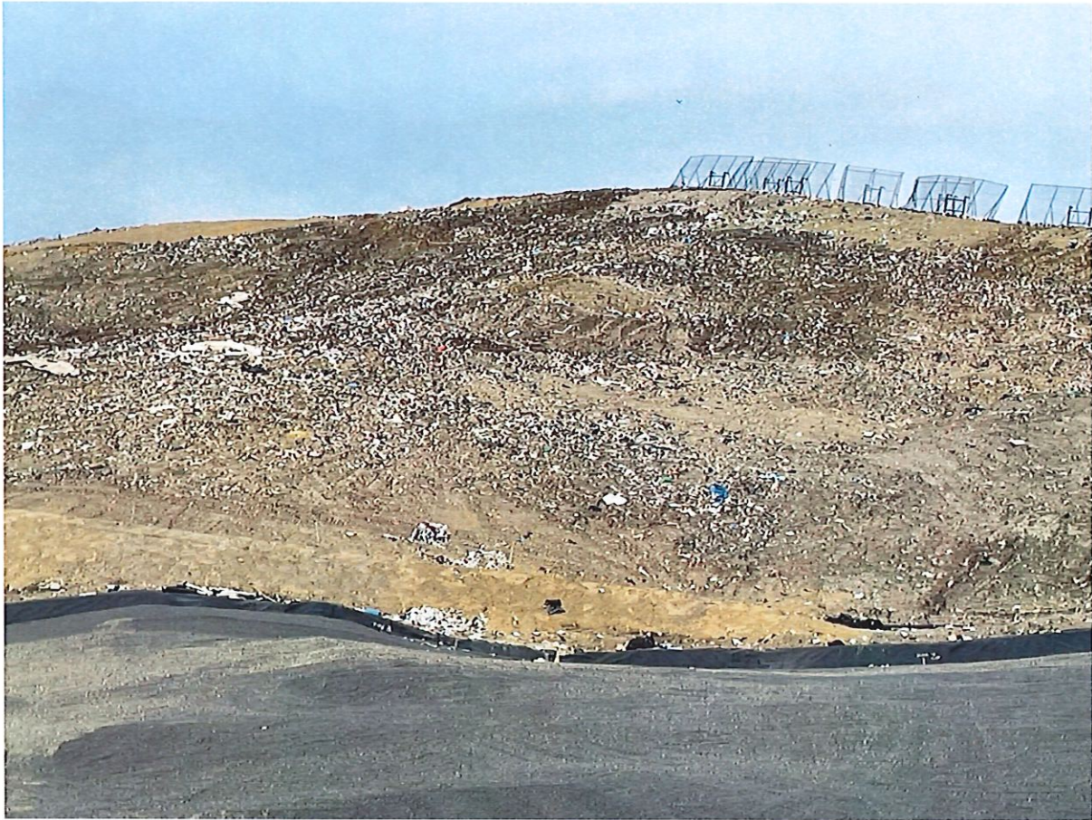
Photo 4: The south slope on the eastern edge of BLC (SE2-AB Phase 1) facing northwest shows exposed and potentially uncompacted waste throughout the disposal area.
