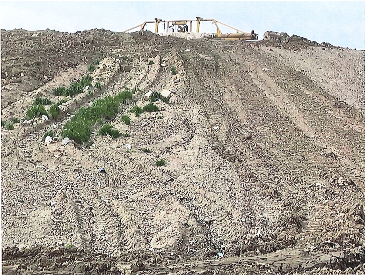
Photo 2: Dozer tracking on intermediate cover on the north slope at BLC.
