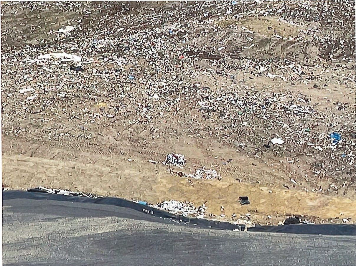
Photo 6: The south slope of SE2-AB shows consistent uncovered waste. An unidentified cube in the foreground was left uncompacted and uncovered.
