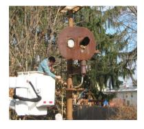
Volunteers from the Saucon Rail Trail Oversight Commission are beginning the first steps in the refurbishment project by disassembling and removing the individual parts of the signal and storing them indoors for the winter. Each part will be photographed, measured, and analyzed to determine if it can be refurbished or will need replacement. This information will be shared with experts who can provide advice and direction on the fabrication, sanding and repainting of the signal equipment.
